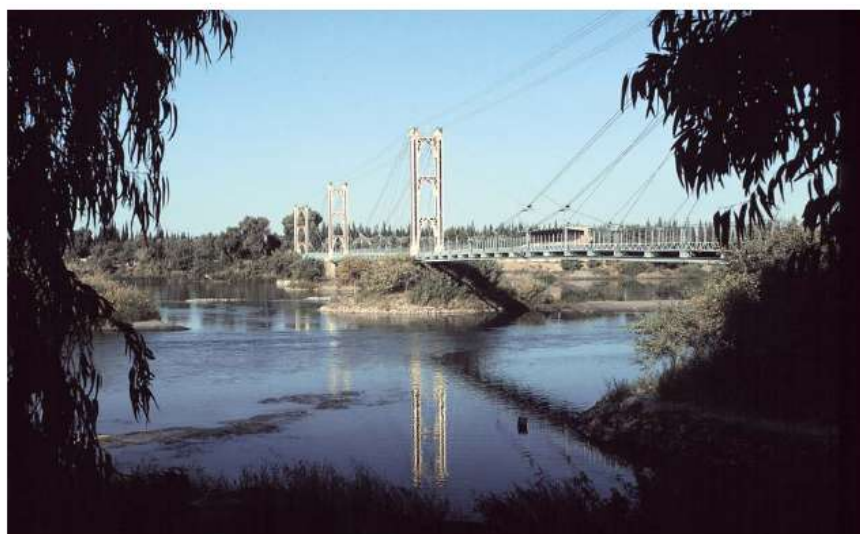
Suspension bridge over Euphrates at Deir El Zore – Syria (Source: UNEP, 2009)
